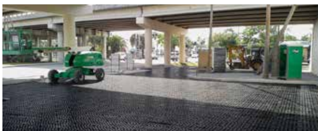
FLODOT UNDERPASS PROJECT
