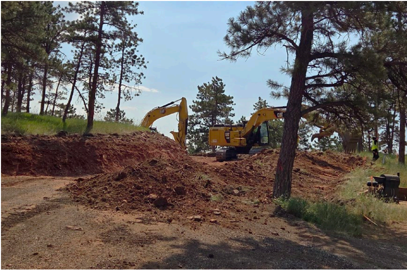
Road improvements have begun at Eagle Campground at Carter Lake.
