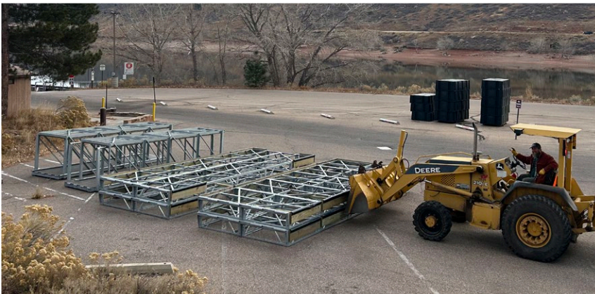
Maintenance crews work on the new docks at Horsetooth Reservoir
